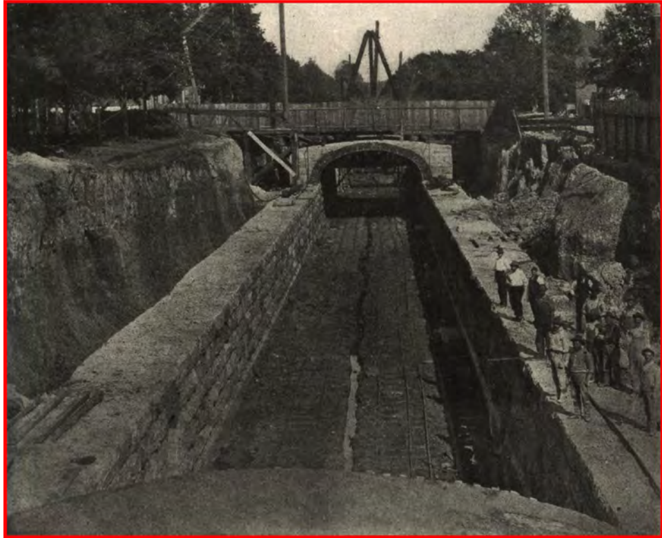
Virginia Avenue Tunnel Construction
