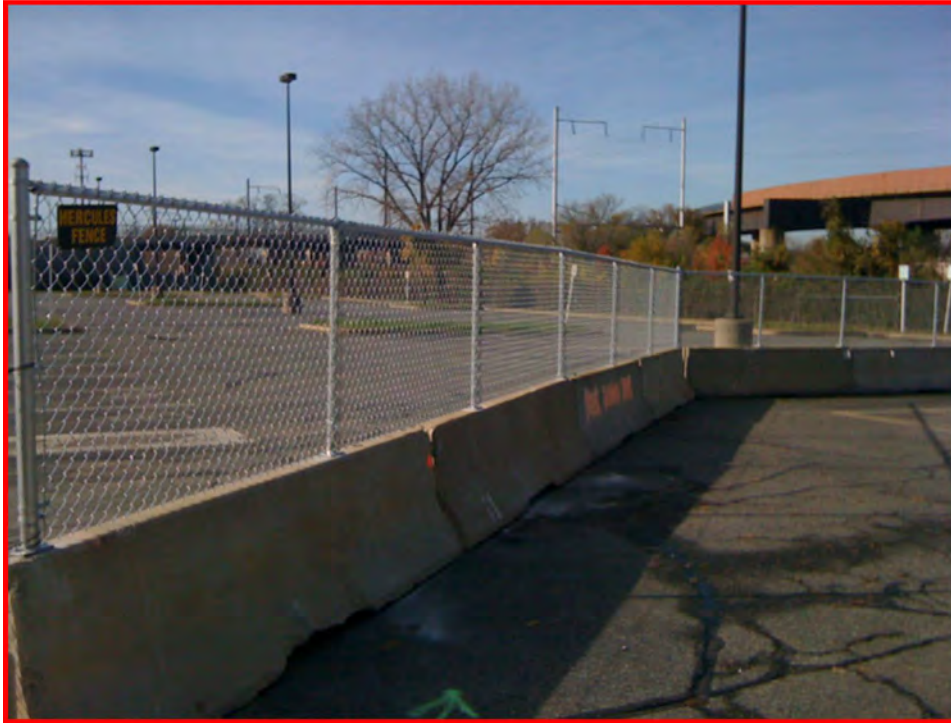
Chain Link Fence Mounted on Traffic Barrier
