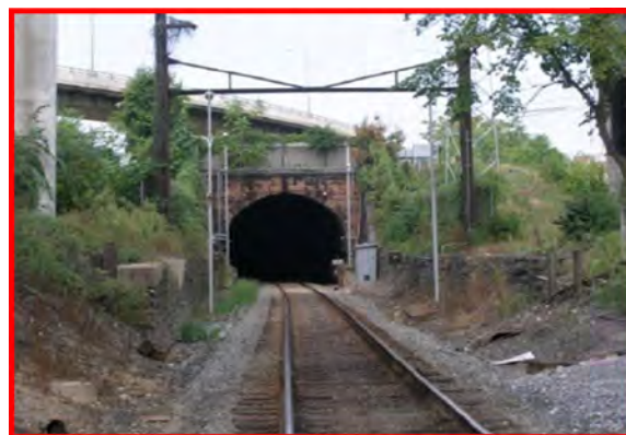
East Tunnel Portal at 11 th Street SE
