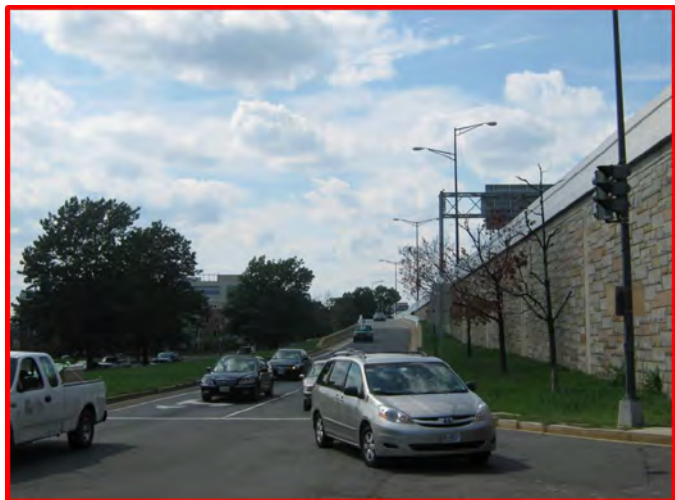
I-695 Off-Ramp at 6 th Street SE
