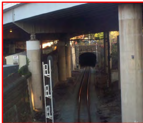
West Tunnel Portal at 2 nd Street SE
