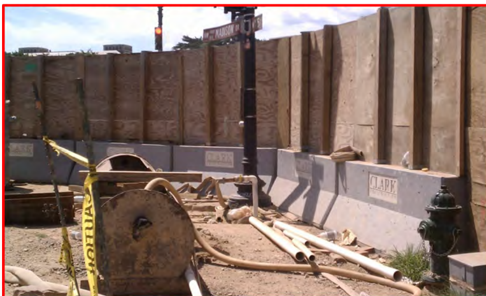
Stockade Fence Mounted on Traffic Barrier
