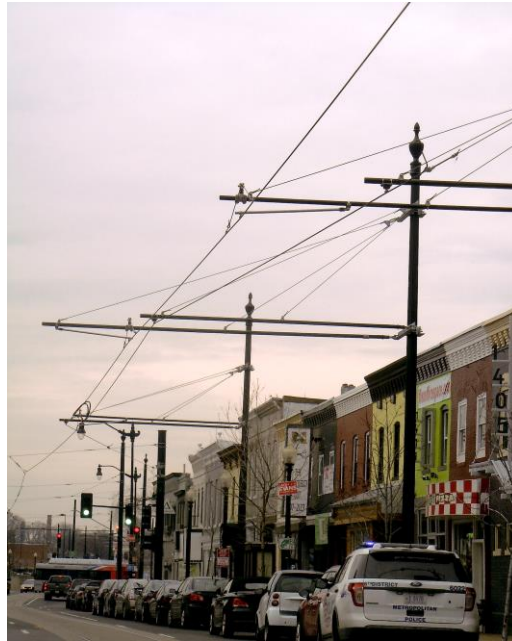
H St. NE – streetcar stanchions and wires – (Photo: Meg Maguire)
