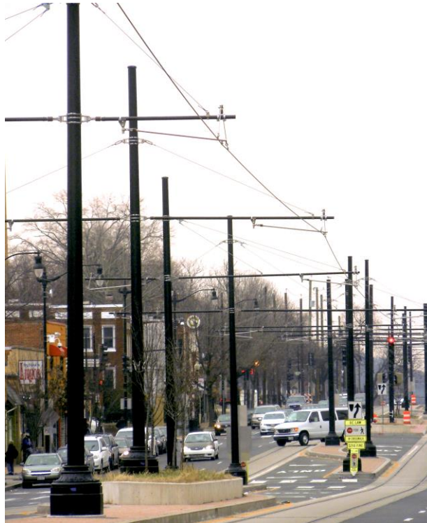
Benning Rd., NE –streetcar stanchions and wires – (Photo: Meg Maguire)
