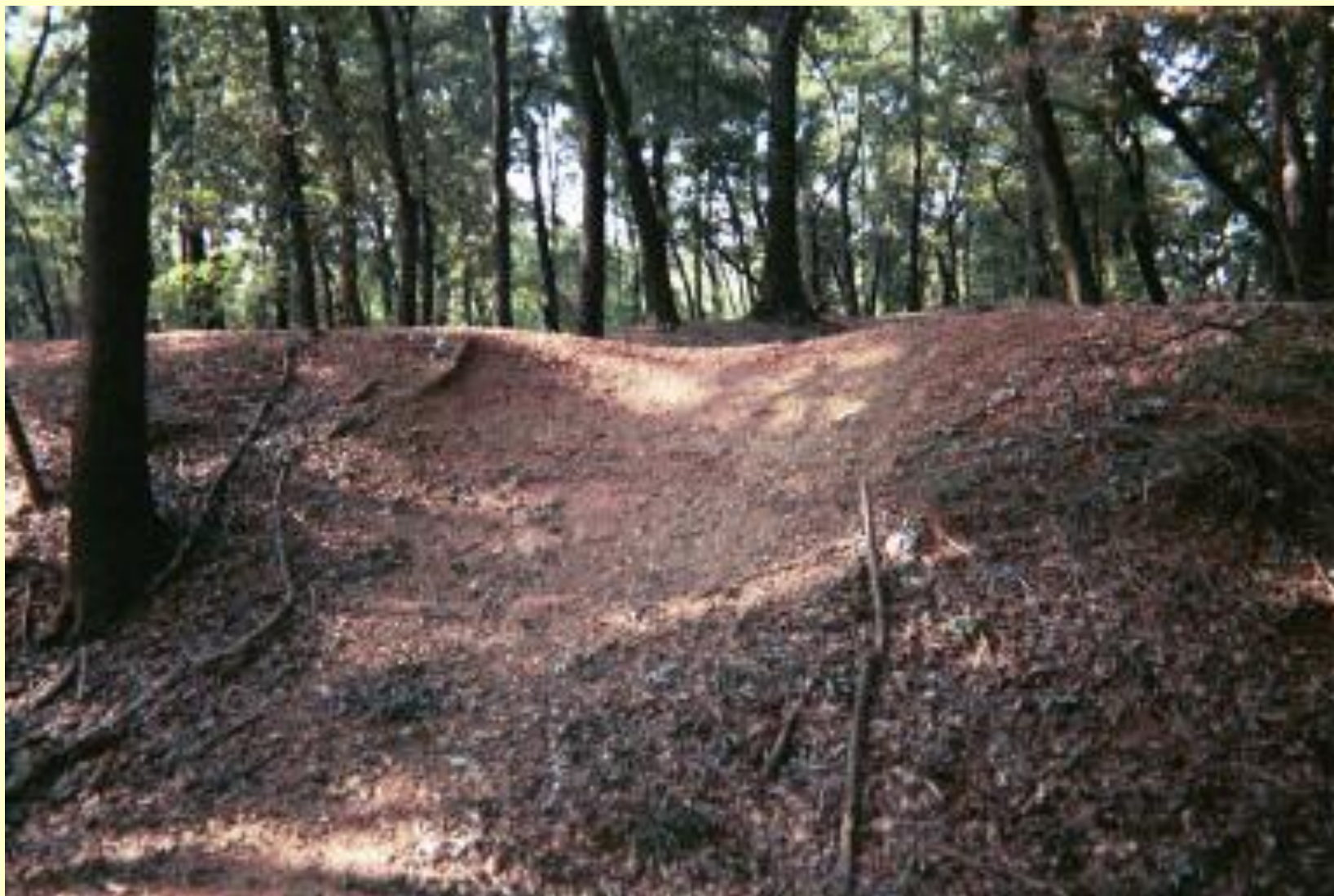
Erosion of Fort Totten Civil War Earthworks from Dirt Bikes
